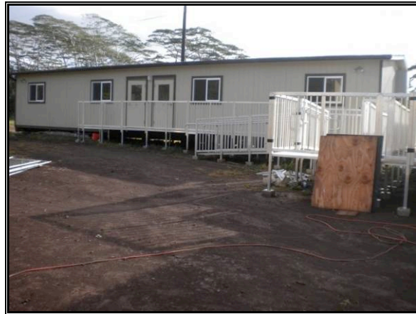
New modular classrooms installed July 2013
