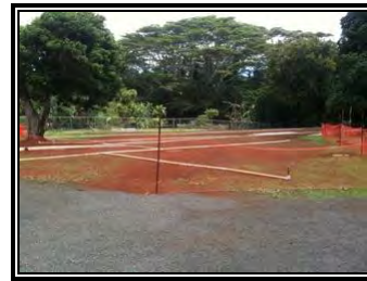
New lawn installation
