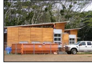
Year 3: Construction Begins
