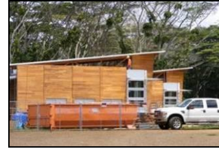
Year 3: Construction Begins
