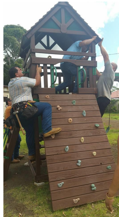
Installing the new playground equipment
