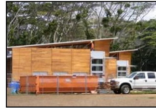
Year 3: Construction Begins
